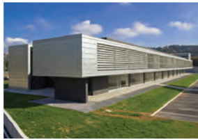
New buildings for the Camerino's University Camerino -Macerata 2008
