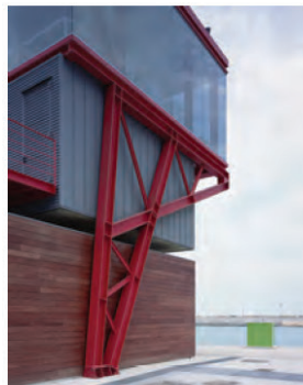
Control tower on the port Marina di Ragusa- Ragusa 2010
