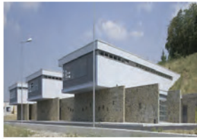
New buildings for the Camerino's University Camerino -Macerata 2007
